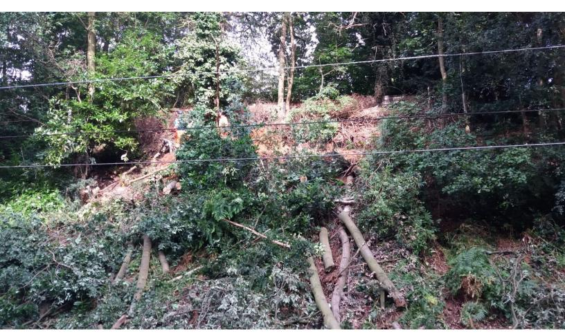
In the last 24 hours, two trees have fallen onto the line, badly damaging overhead power lines, and a section of the embankment, north of University station, has become unstable.
