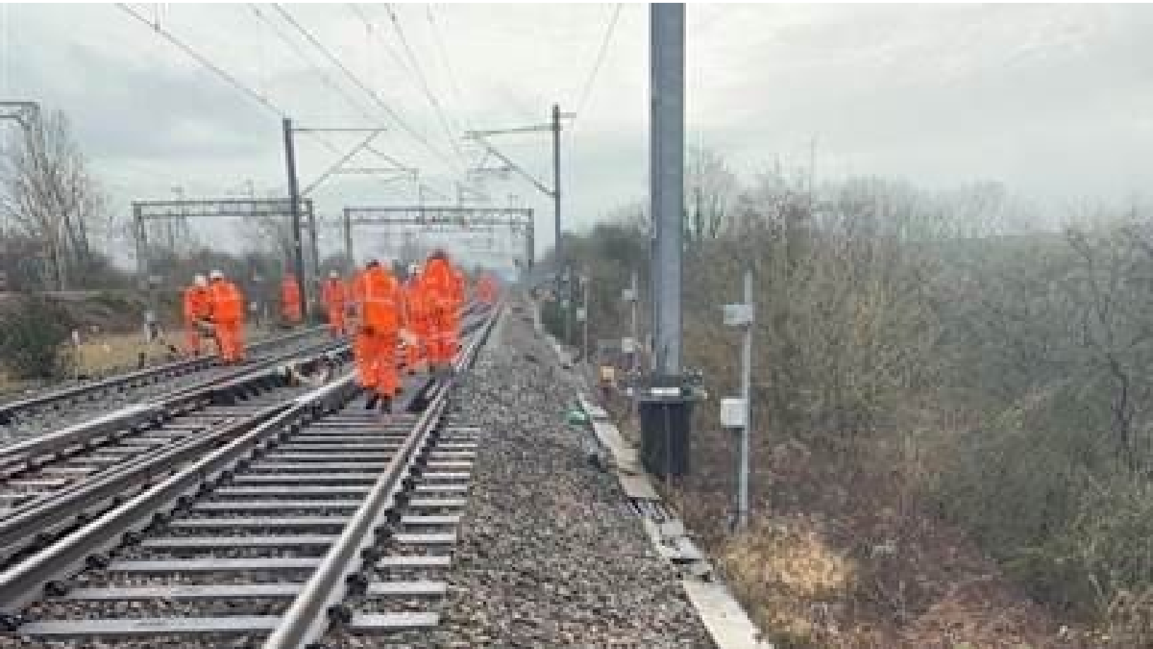
Network Rail engineers on site at Hillmorton
