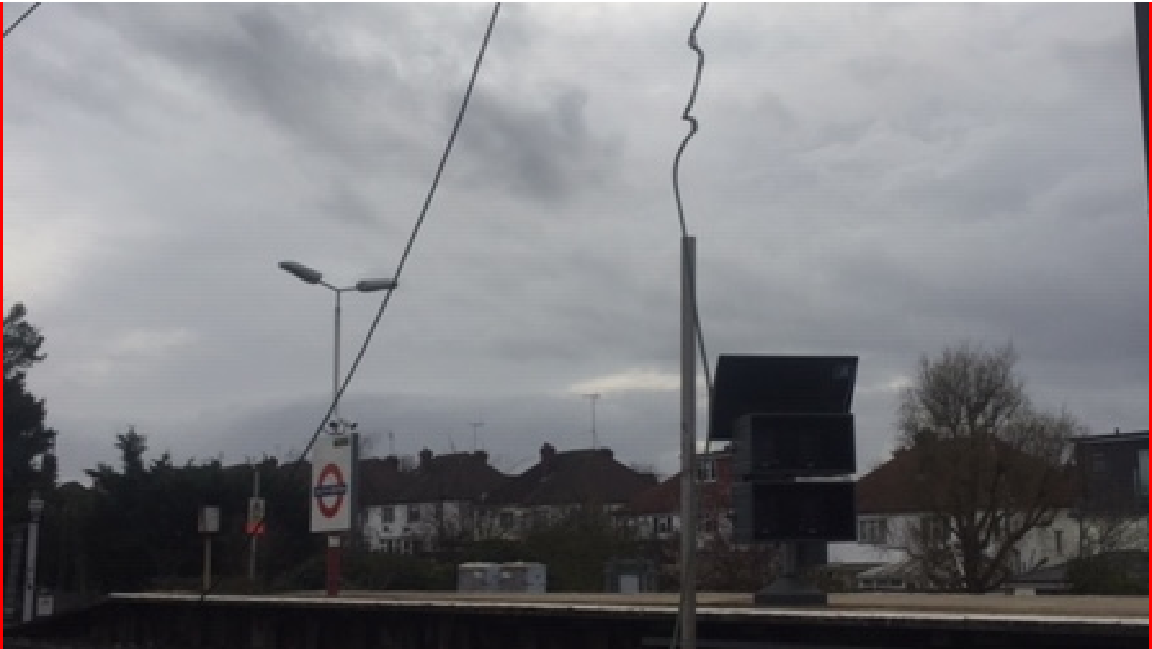
Damage to overhead power lines outside Euston
