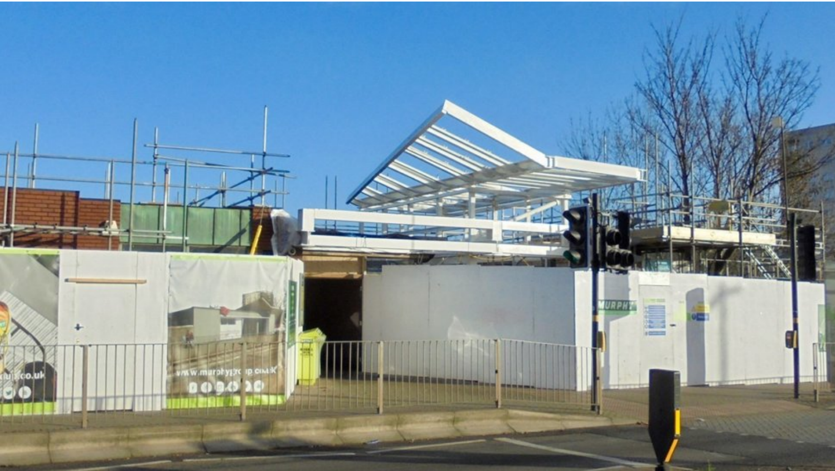
Work is ongoing at Longbridge station
