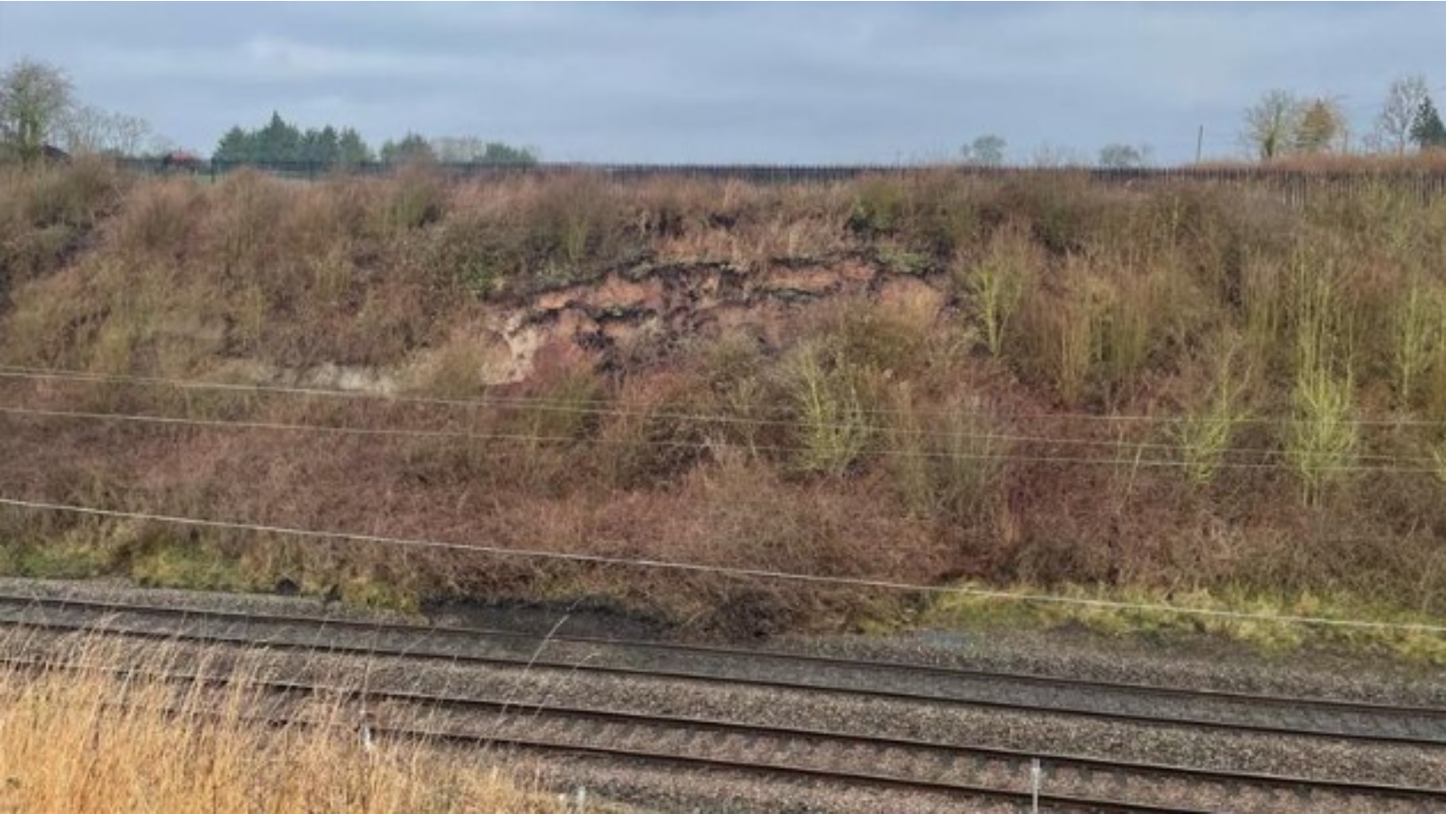
The landslide at Church Lawton, in Warwickshire
