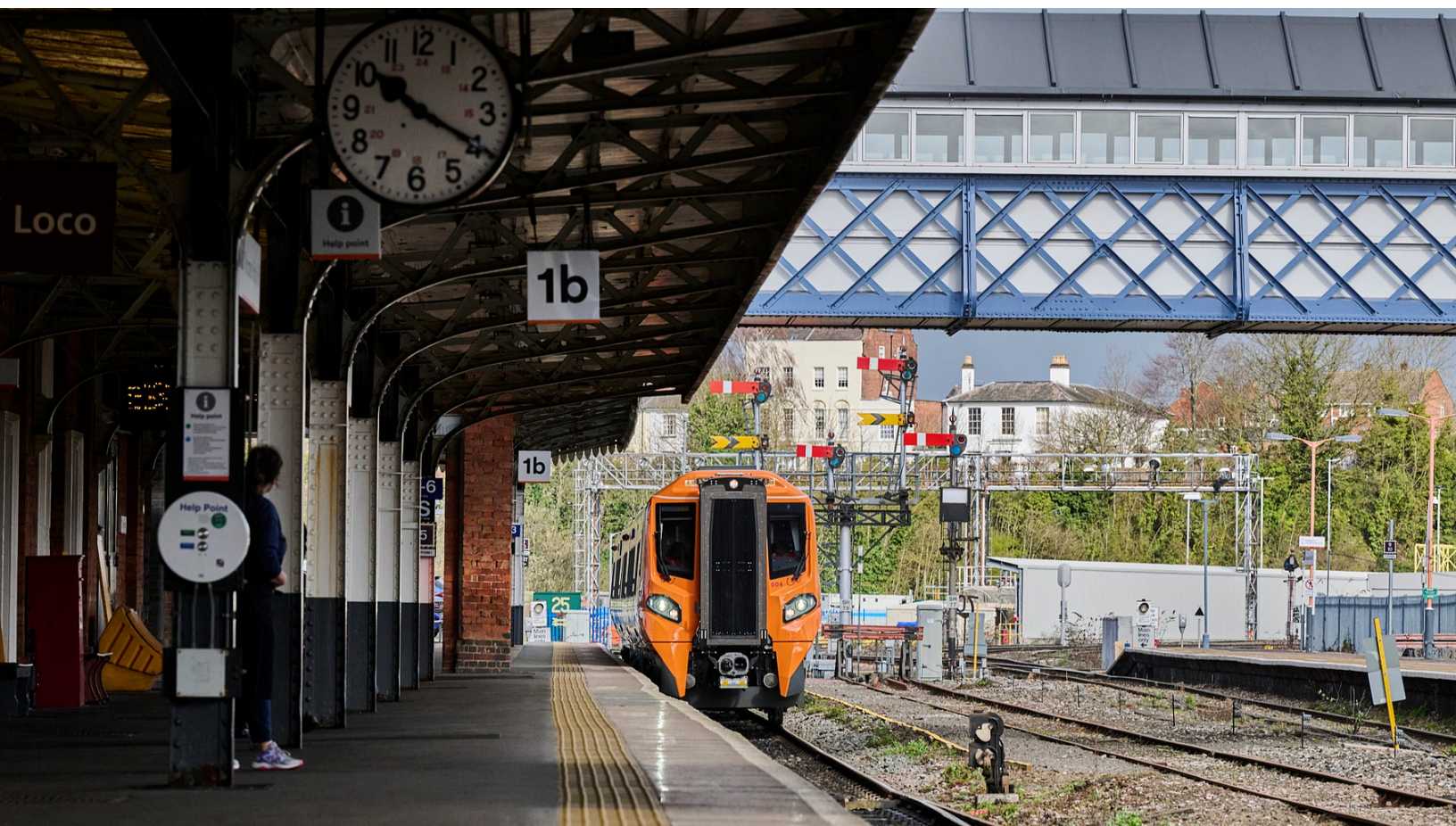
Worcester Shrub Hill station, platform 1b
