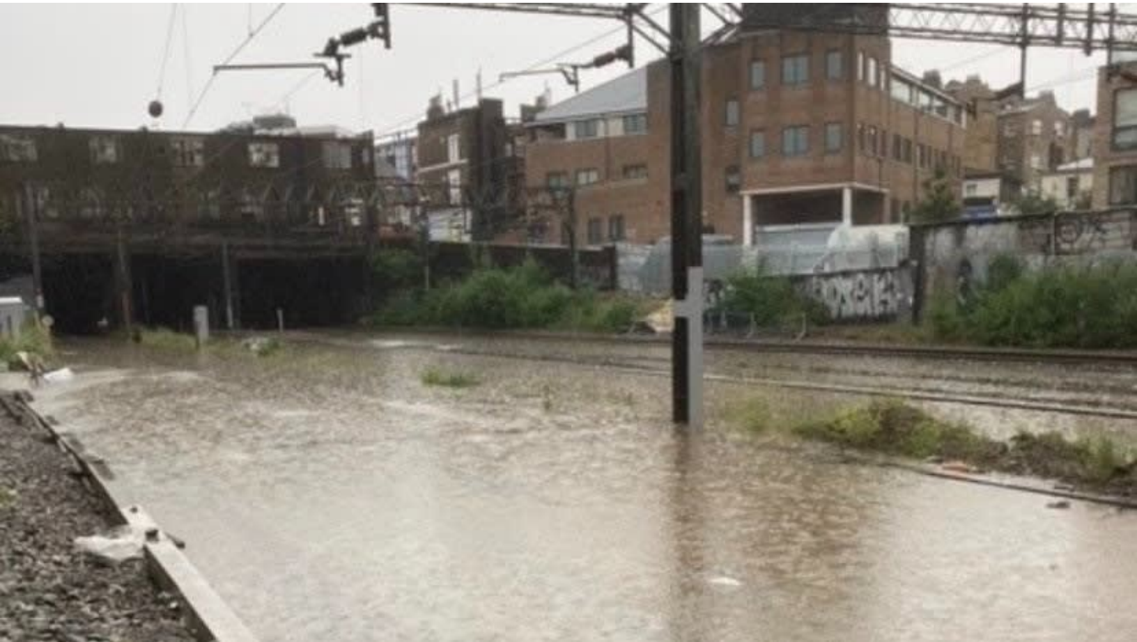
Flooded Track outside Euston Station Monday 12 July 2021
